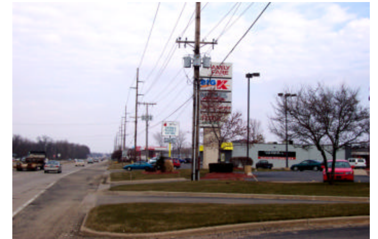
Unsightly Overhead Power lines on Chicago Drive
